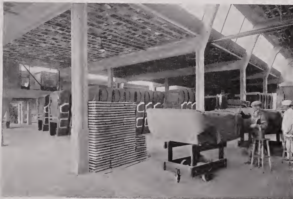
PUTTING ON THE FIRST COAT
